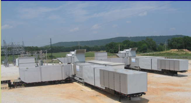
Globex was contracted to Engineer, Package, and Install 2 complete Gas Turbine Powered 20 MW (each) Peaking Plants
